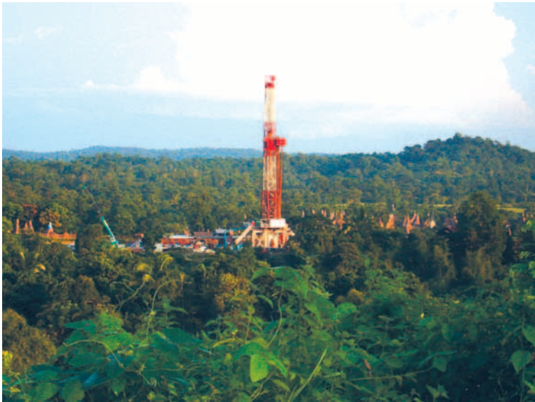
An overview of the drilling rig at Renandaung
